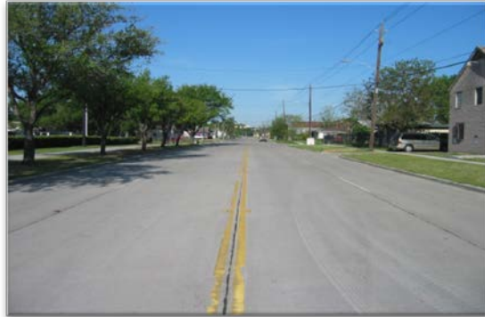
Market Street Reconstruction Houston, TX.
