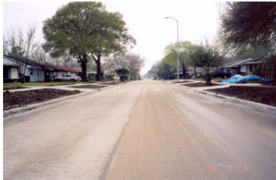
Neighborhood St. Reconstruction Houston
