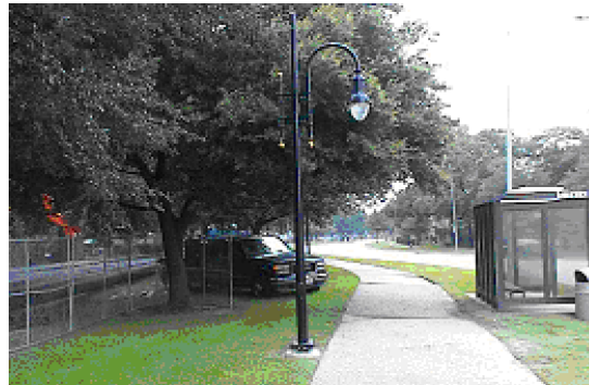
Texas Southern University Campuswide Infrastructure, Houston, TX
