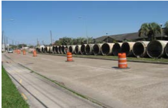
Kirkwyn/Sagemont Drainage Improvements Houston
