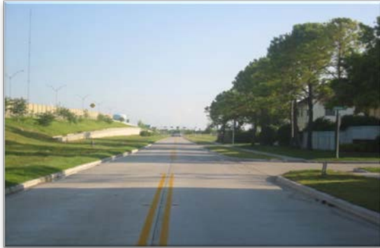
Hillcroft Boulevard Reconstruction Houston, TX.
