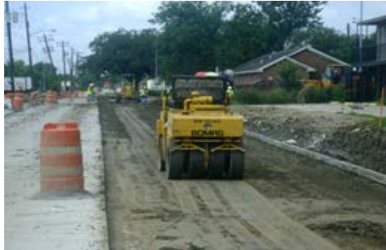
Deats Road Reconstruction Dickinson, TX.
